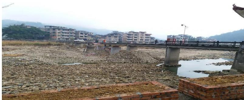
Figure 5: Bridge with River Course Temporary Diverted
